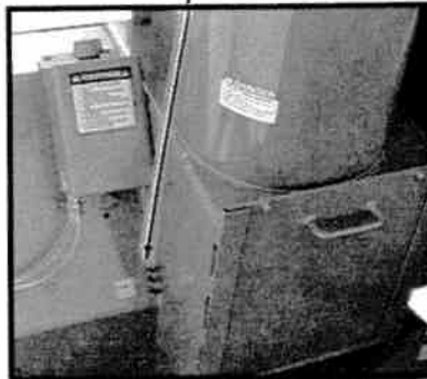
Lower Bearings (Vertical Auger) Front Bearing (Horizontal Auger)
